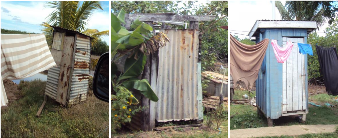
Figure 4: Types of lavatories in Namara squatter settlement.
